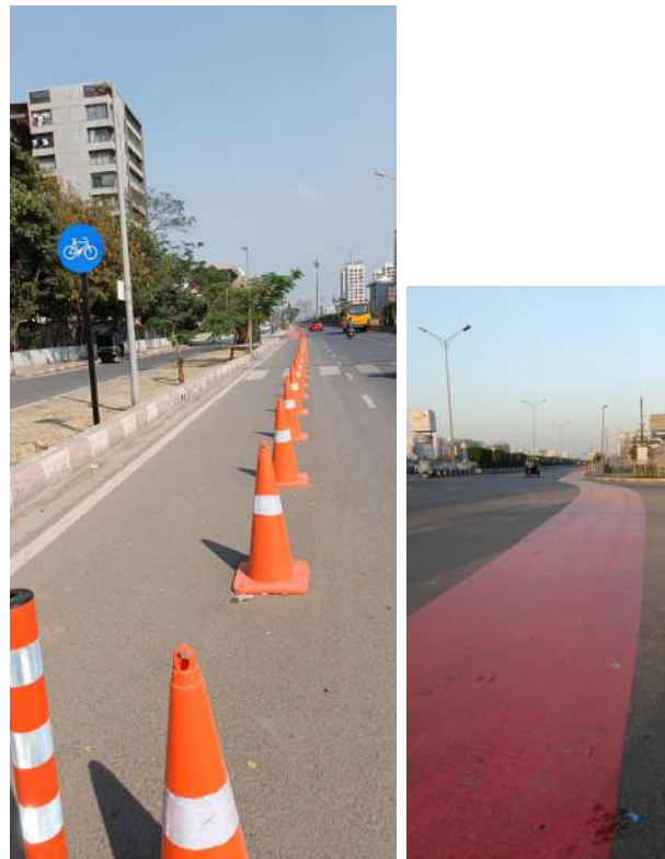
Cycle lanes marked using traffic cones and paint
